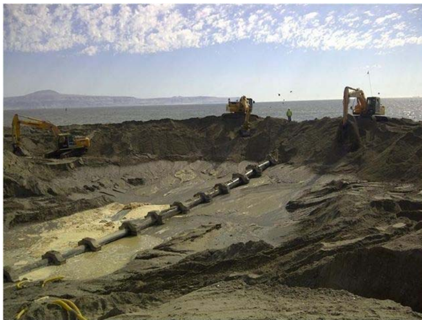
Figure 1 - The construction of Algorta Norte's underground seawater pipeline. (Source:Mch.cl)
