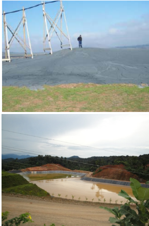
Figure 1 – Thickened (on top) versus traditional tailings (on the bottom). It is possible to appreciate how solid “thickened” ones are. The one on the right instead, has clearly a large content of water. (Source: Galaz, 2011; Minera Petaquilla, 2012)
